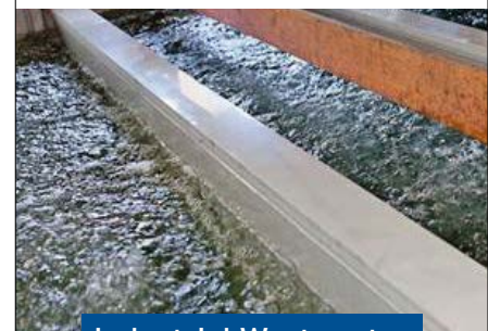
Industrial Wastewater Treatment
